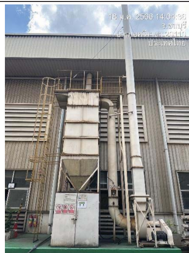
Dust Collector G.8 Forging 3
