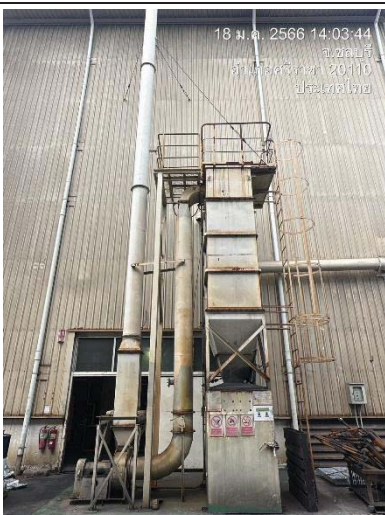
Dust Collector G.8 Forging 2
